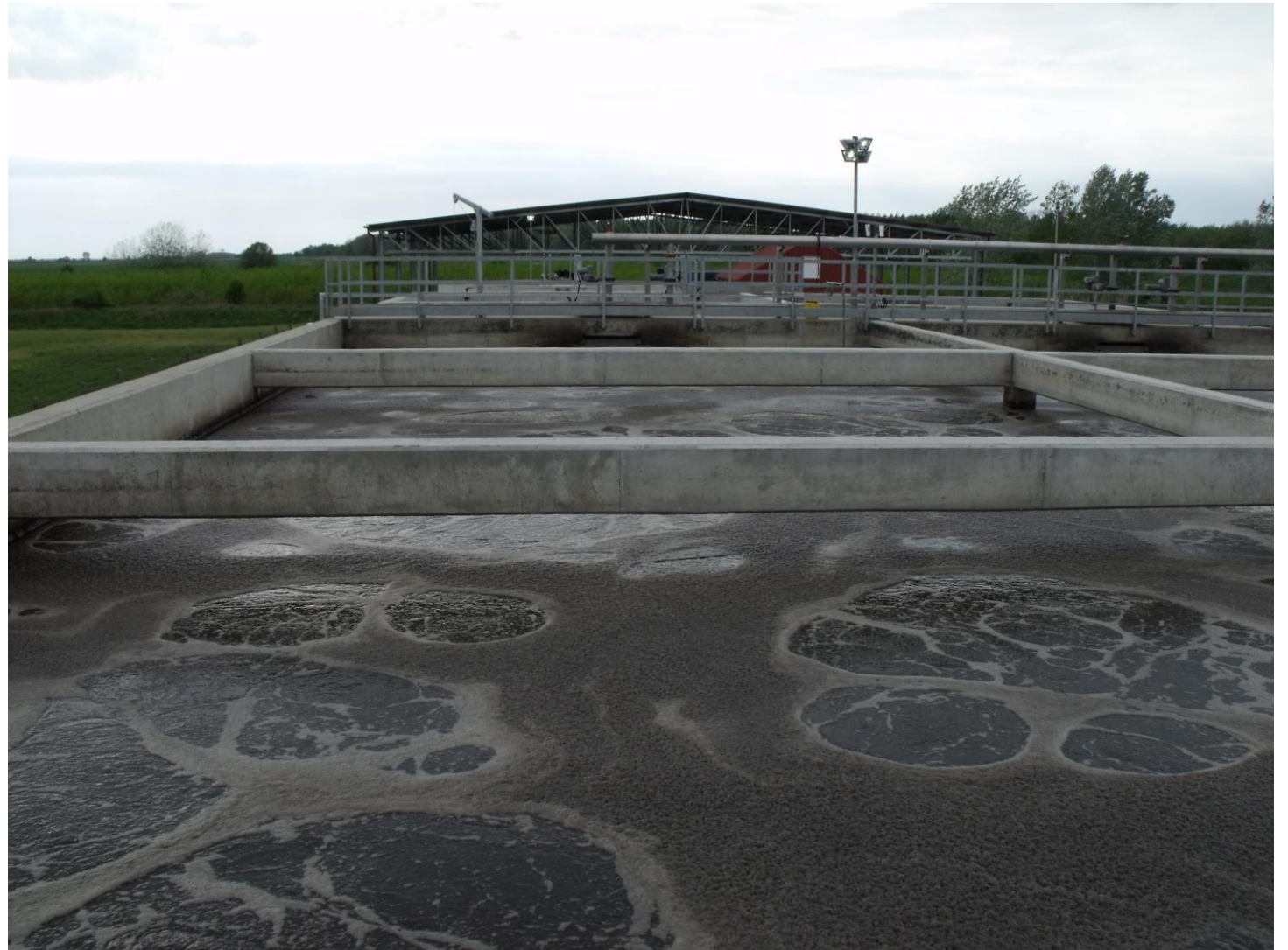
Mechanical pre-treatment unit, biological treatment (BIOCOS technology), sludge thickening, disinfection
